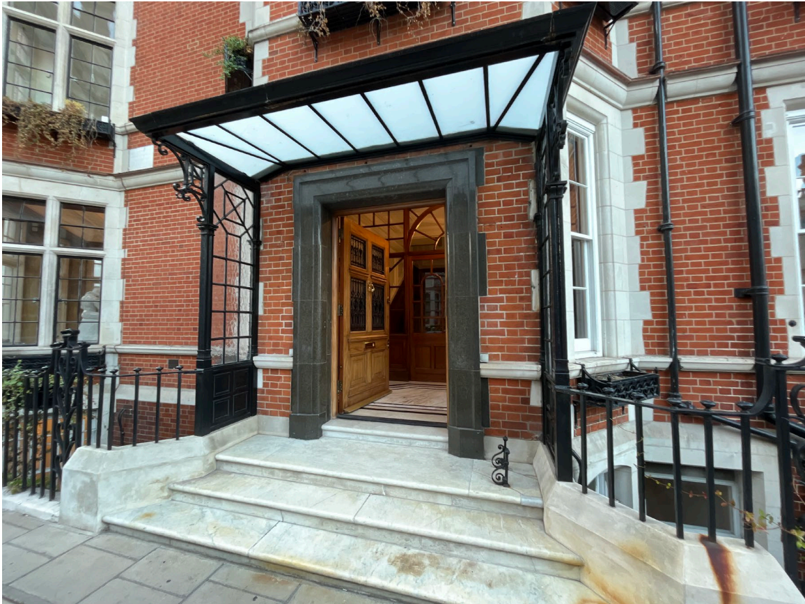
1. The main entrance to the proposed premises on Aldford Street.
